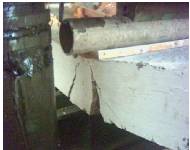
Figure 4: Failure mode of slab models under loading.
